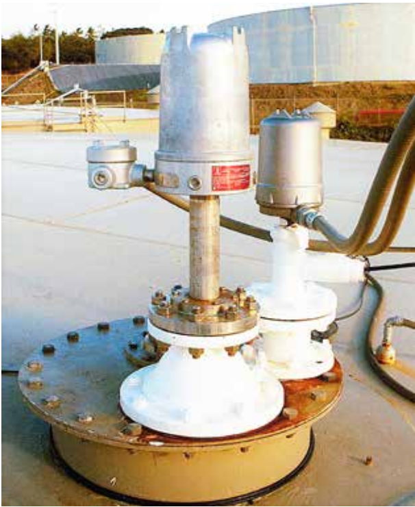
Figure 2. Advanced hydrostatic gauge with multiple pressure and temperature sensors installed in a single 2 in. tank penetration. Also shown is an independent high level alarm switch for overfill protection.
