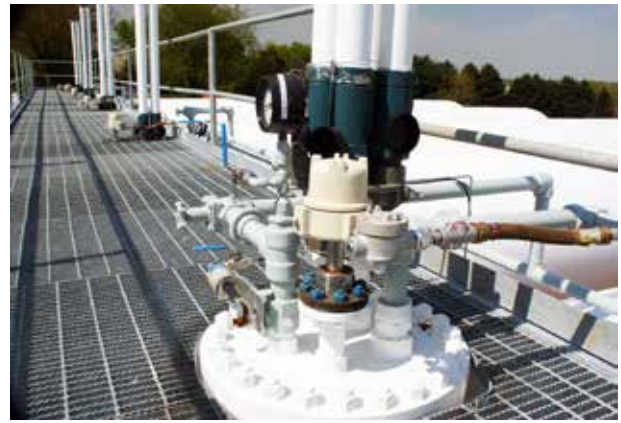
Figure 3. Multi-section advanced capacitance gauges with multiple capacitance and temperature sensors installed in a battery of horizontal tanks.
